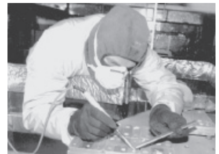
Application of Filler to Cold Commissioning Model
