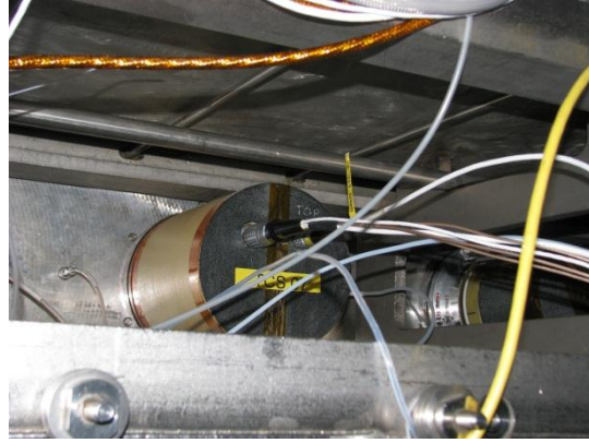
Figure 5: Camera installed in the Top-Wall
